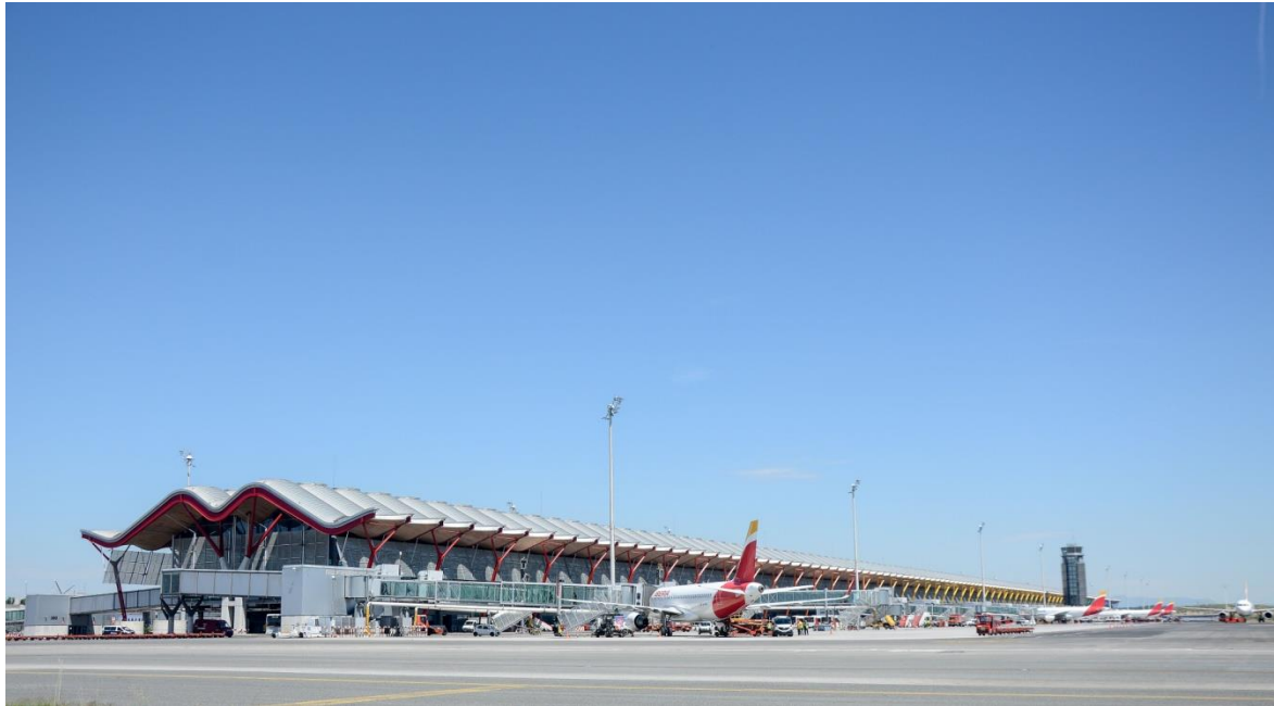
Figure 4.7 Adolfo Suárez Madrid-Barajas Airport state-of-the-art facilities
