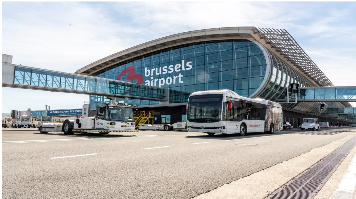
Figure 5.1 Brussels Airport modern state-of-the-art infrastructure facilities
