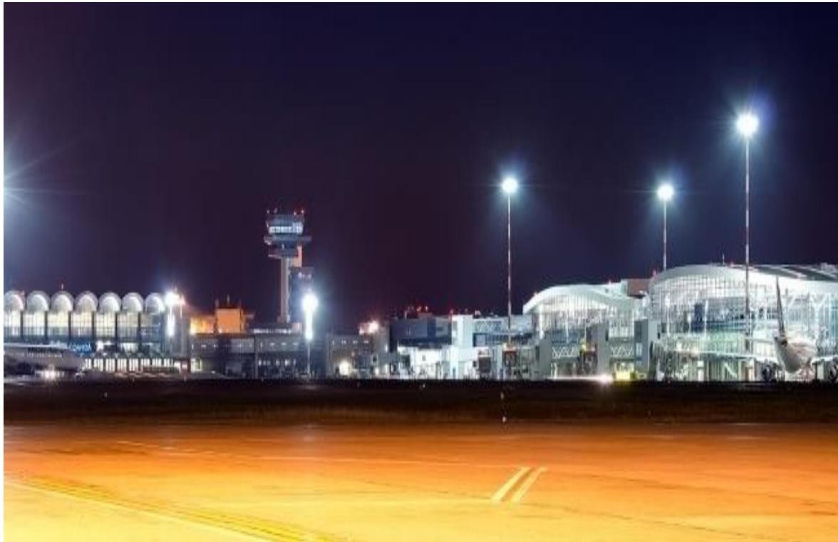
Figure 5.10 Bucharest Henri Coandă International Airport world class infrastructure facilities
