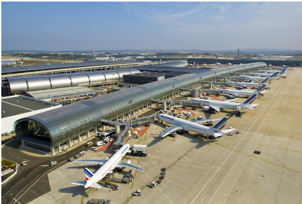
Figure 4.9 Paris-Charles de Gaulle Airport astounding world class climate friendly infrastructure facilities
