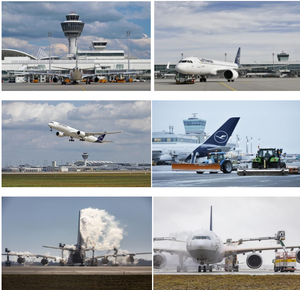
Figure 2.27 Munich Airport modern technology (deicing of snow/ice) equipment and facilities
