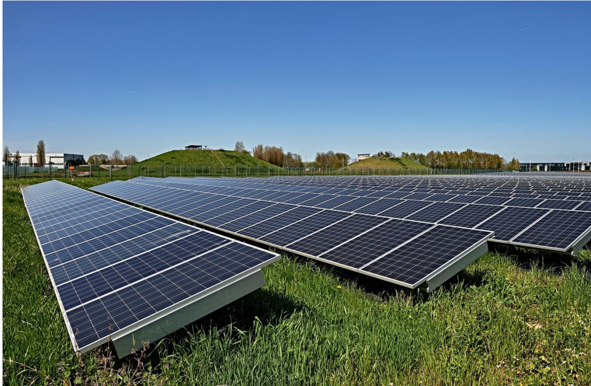
Figure 5.2 Brussels Airport globally recognized eco-friendly infrastructure facilities
