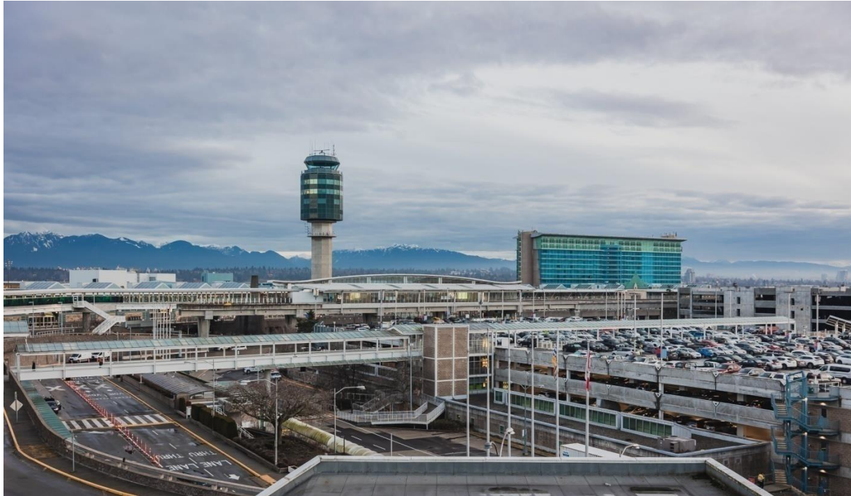
Figure 2.20 Vancouver International Airport – YVR modern infrastructure facilities
