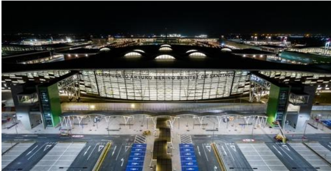
Figure 3.16 Arturo-Merito Benítez International Airport astounding night view
