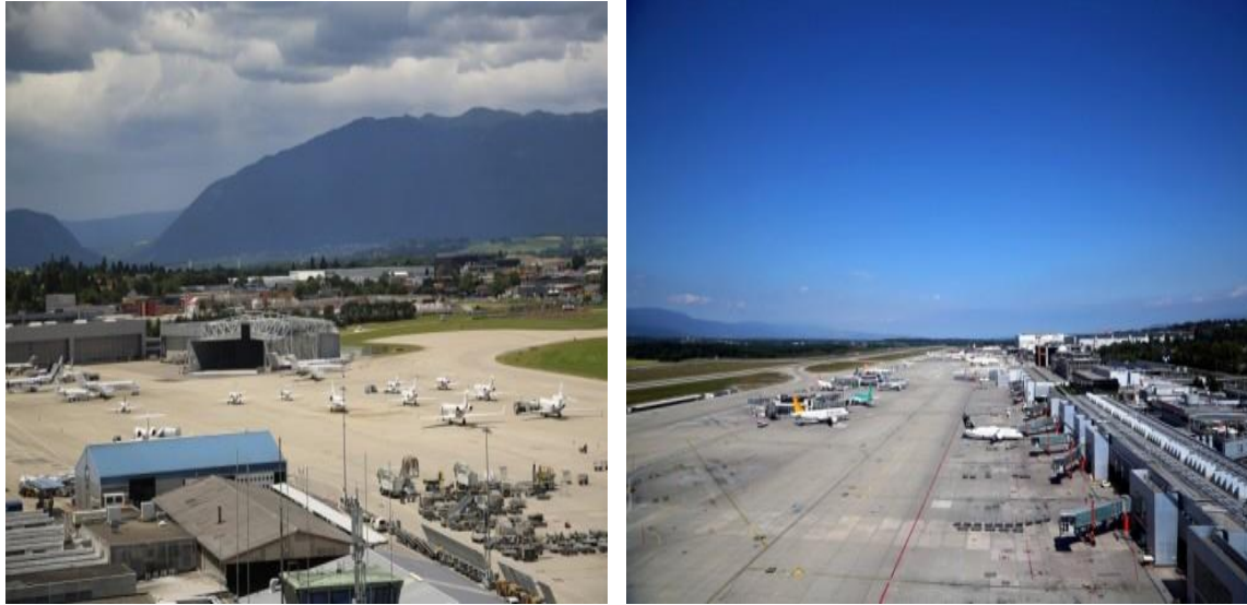
Figure 2.10 Genève Aéroport world class tarmac and runways infrastructure
