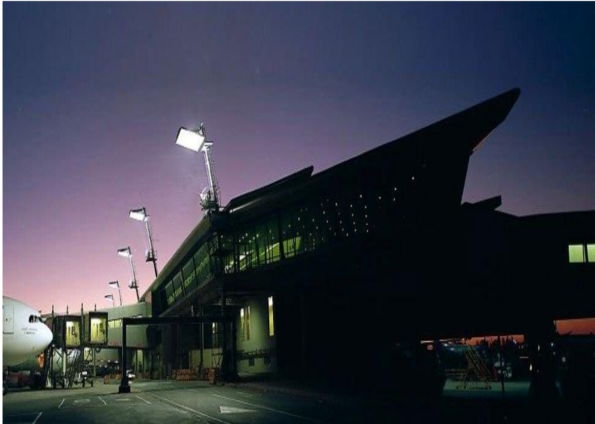
Figure 3.13 O.R. Tambo International Airport state-of-the-art facilities
