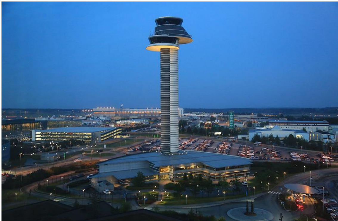
Figure 4.17 Stockholm Arlanda Airport world class infrastructure facilities
