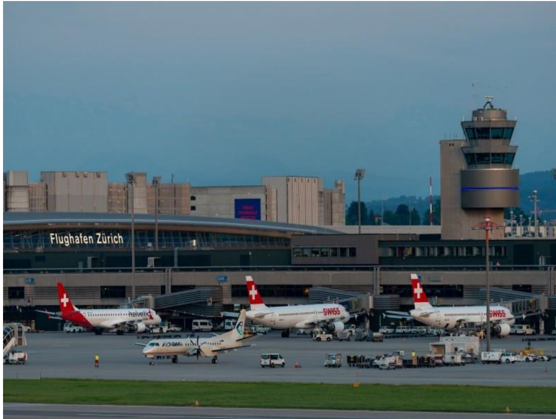
Figure 2.2 Zurich Airport outside infrastructure facilities
