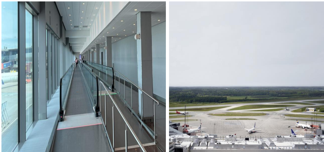
Figure 4.16 Stockholm Arlanda Airport passageway, aircraft stands & parking spaces facilities
