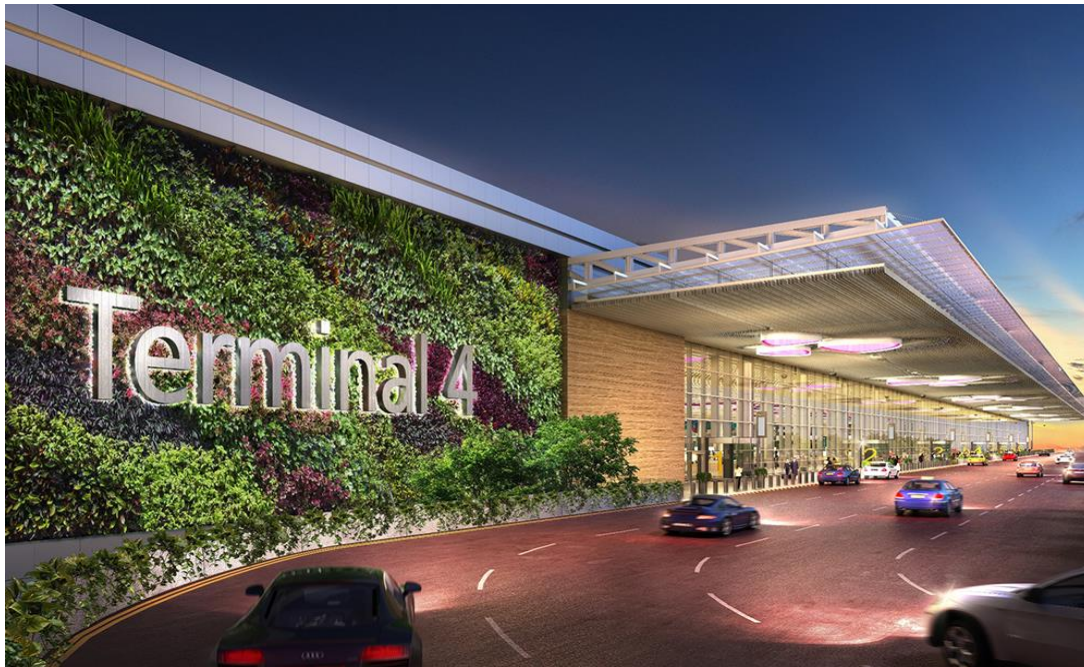
Figure 4.5 Changi Airport Terminal 4 infrastructure
