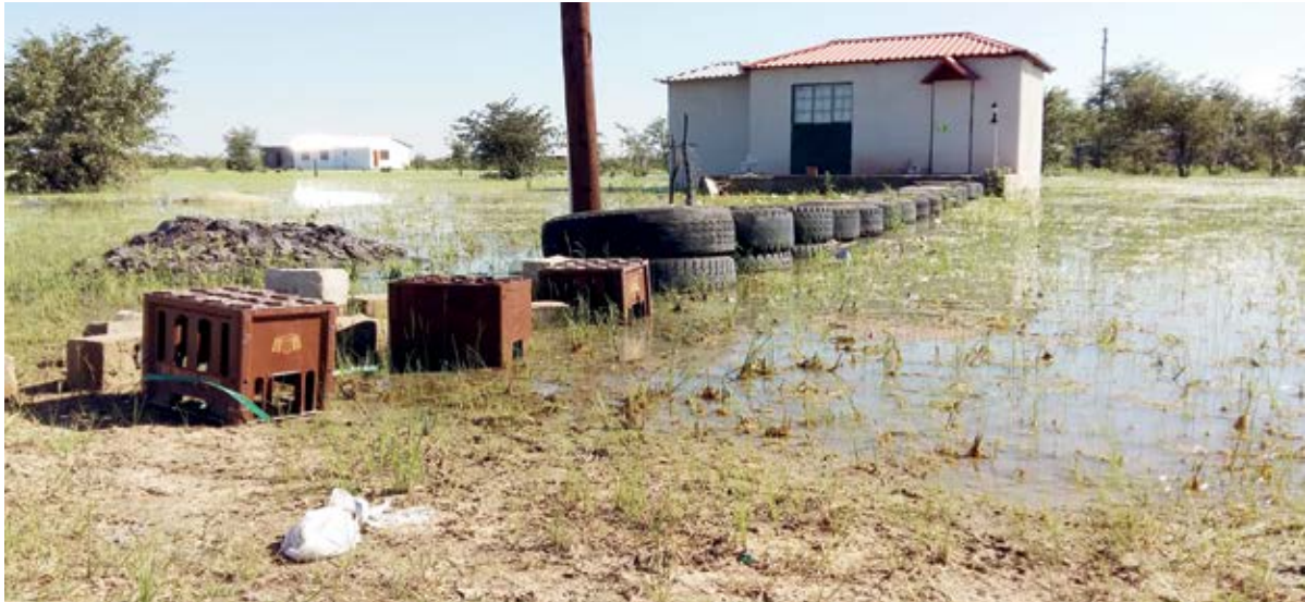
Figure 30: An example of modification of the surroundings to cope with flooding. In this case, old tyres and crates were used to facilitate access to the buildings during the flooding. The effectiveness of this rudimentary modification in the case of extreme floods is not known.
