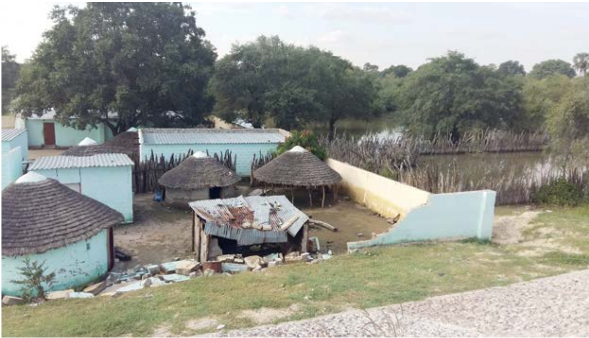
Figure 27: An example of a homestead damaged by flooding induced by the newly developed road near-by the homestead in the Cuvelai Basin. Note the water marks on the inner wall of the homestead.
