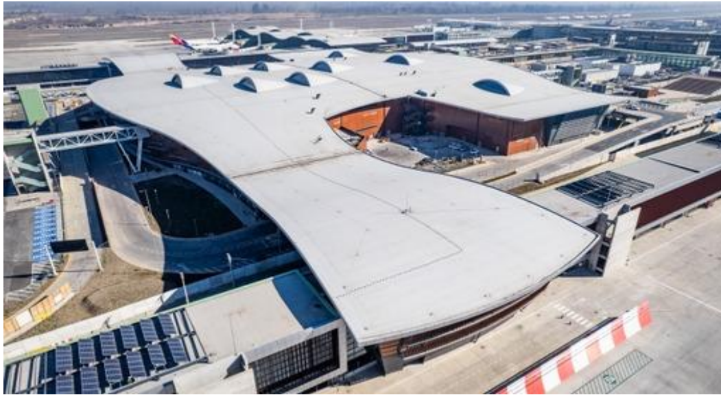
Figure 3.21 Arturo-Merito Benítez International Airport infrastructure development
