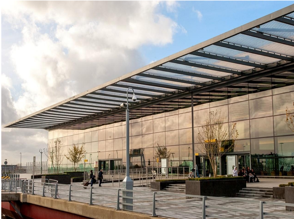
Figure 3.9 London Heathrow Airport Terminal 4
