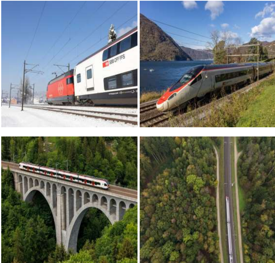
Figure 8.2 The state-of-the-art astounding exterior features and aerial views of the trains owned by SBB
