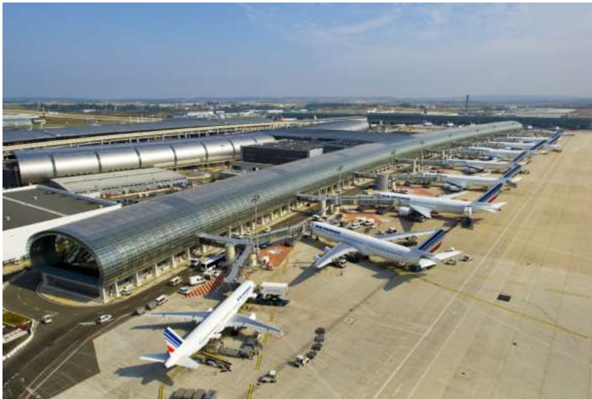
Figure 6.9 Paris-Charles de Gaulle Airport astounding world class climate friendly infrastructure facilities
