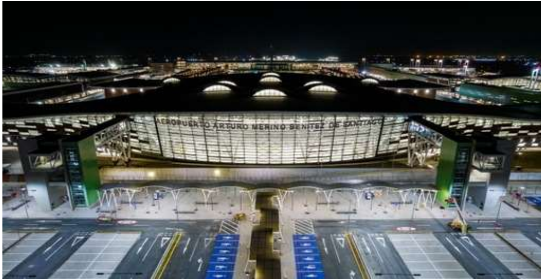
Figure 6.3 Arturo-Merito Benítez International Airport astounding night view
