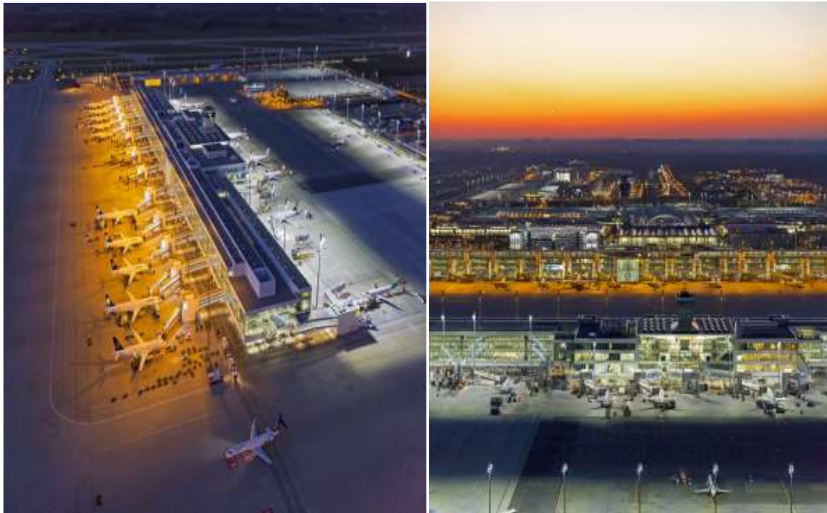
Figure 6.18 Munich Airport’s state-of-the-art aircraft arrival terminals infrastructure
